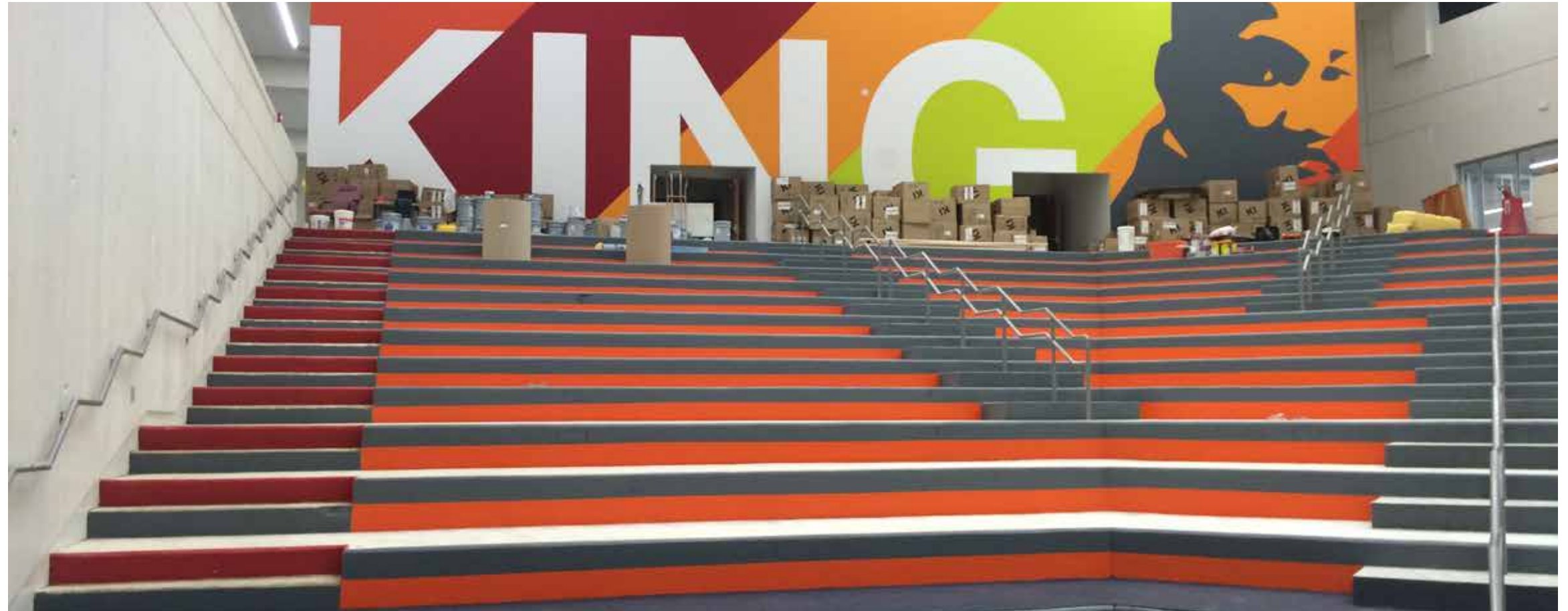
King Middle School under renovation, Atlanta, GA.
