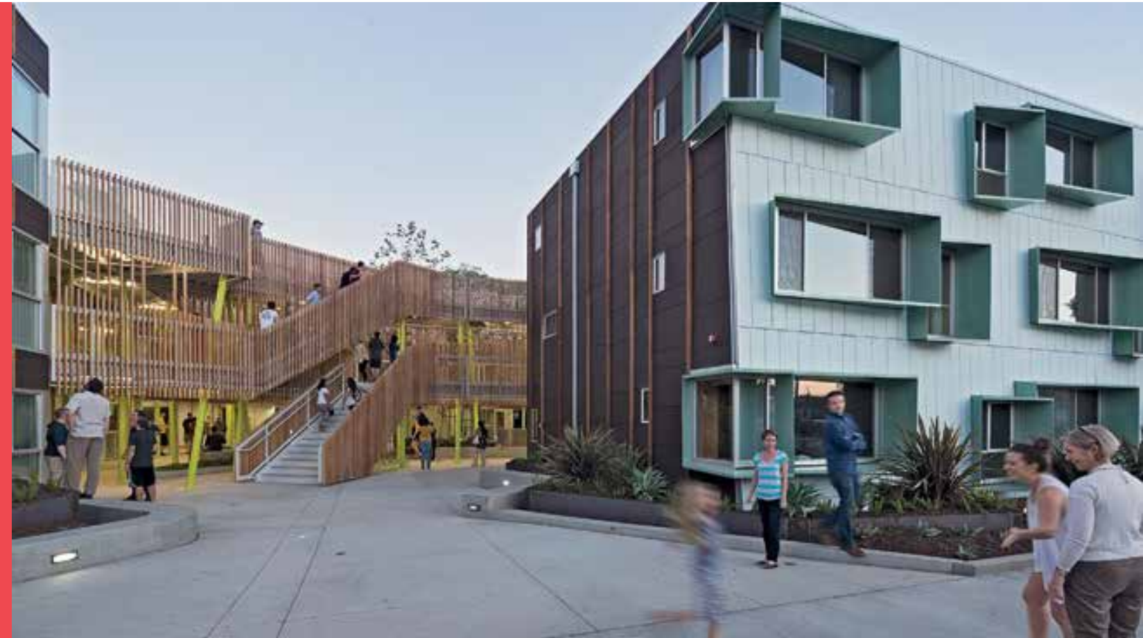
2602 Broadway - Affordable housing building. Santa Monica, CA.
